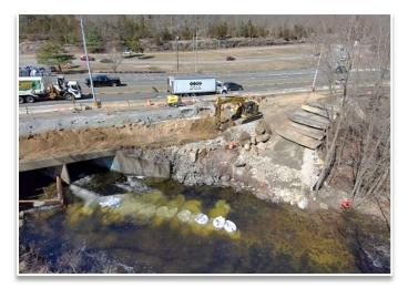
These modifications will allow for retaining walls to be constructed on either side of the culvert, both northbound and southbound, to increase the width of I-95 and improve driving safety in this area.
